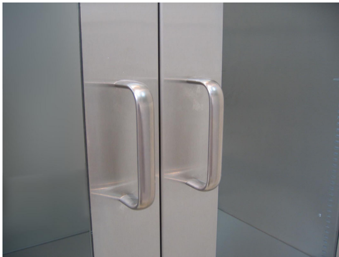
Solid stainless steel handles. Nylon roller door catches.
